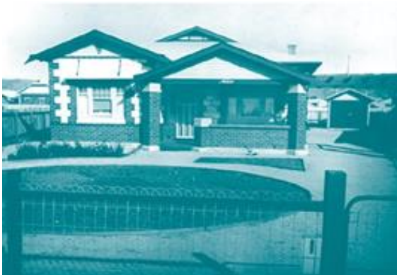
Traditionally garages were located at the end of the driveway. This one car garage was located at Ludgate Circus.
