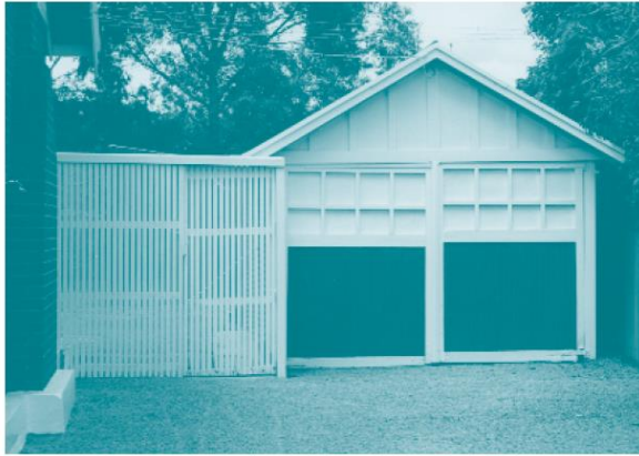
This early garage is still standing in Ludgate Circus. Note the use of sliding door.
