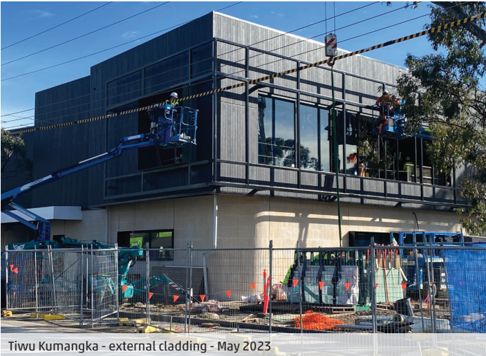
Tiwu Kumangka - external cladding - May 2023
