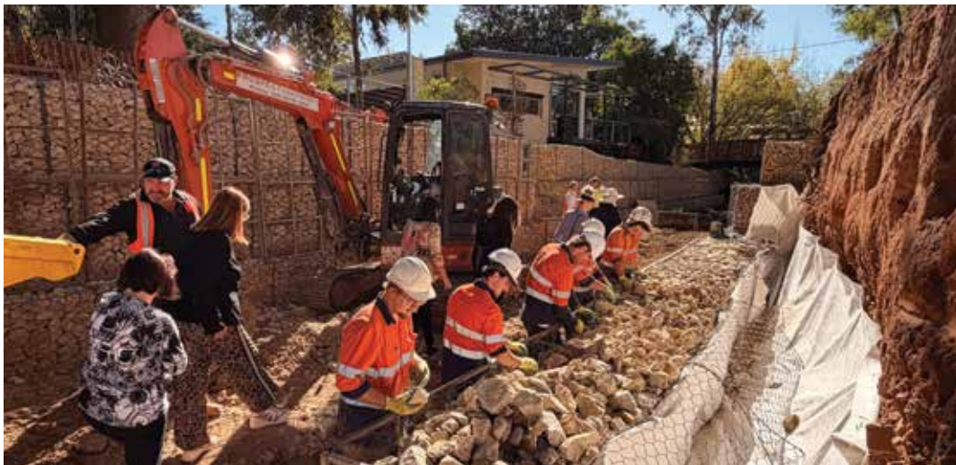
Gabion walls have been installed at Betty Long Gardens, Torrens Park, to prevent erosion and flooding.
