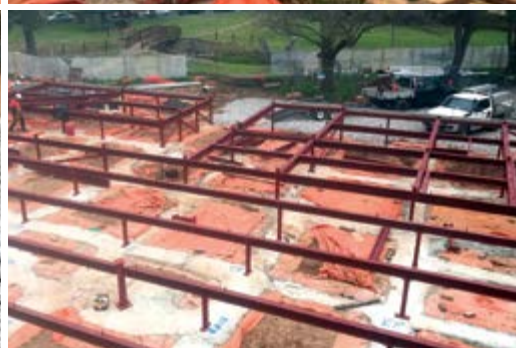
Clockwise from top left: Concrete footings; Hydraulic underground services; Permeable paving to car park; Steel in the suspended slab.
