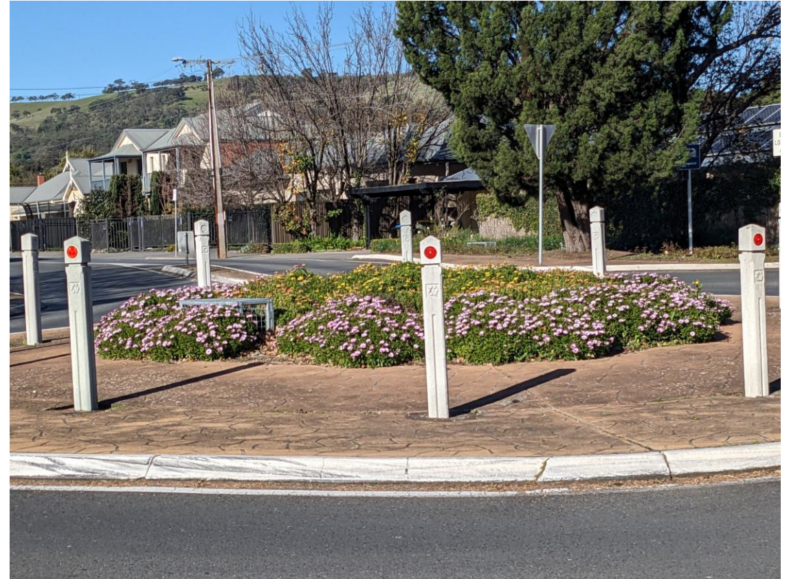
Pictured: Ayr Ave / Princes Rd irrigated roundabout protected by recycled bollards and caged meter box
